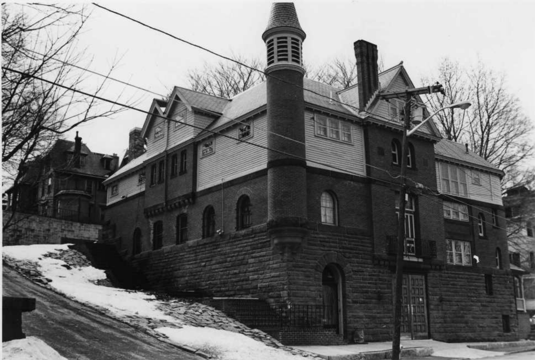
2. View looking southwest at 579 E. Merrimack St. (foreground) and 396 Andover St. (rear). (Photograph: Elizabeth Durfee Hengen, July 1983)
