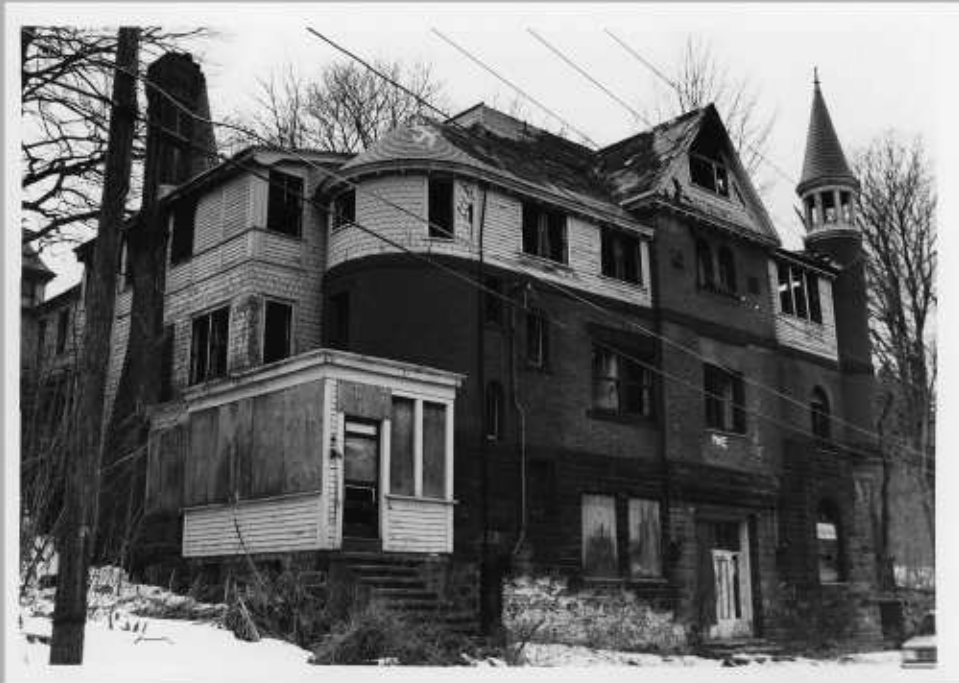
3. View looking southwest at 569 E. Merrimack St. (Hoyt Carriage House)
