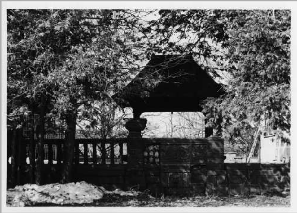
4. View looking north between the Hoyt and Shedd Houses at gazebo.
